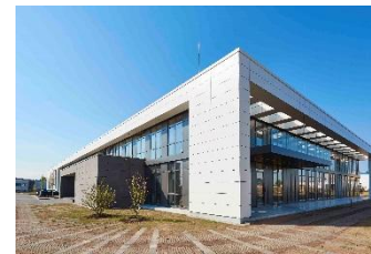
Elementar moves into new headquarters in Langenselbold near Frankfurt, Germany
